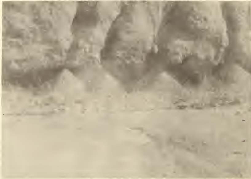
Figure 8.--The canes of loose soil are the result of freezing and thawing on a 1:1 Cecil clay unprotected roadbank facing north. The loose soil rolled down the bank into the ditch in a 2-day period after thawing.
